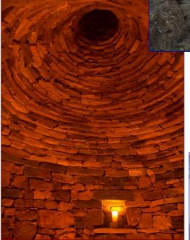
Here again alcoves were built into the walls, this time to allow for lighting.
