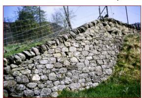
The copes are placed carefully on steps created as the wall is constructed.
