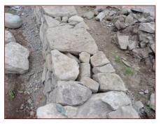
During a training course the students look sceptical when I tell them that I spend half my working time doing hearting. It is essential, as with poor hearting the wall will collapse in or fall out. The spaces underneath and between the building stones should be filled first with the largest non-building rocks which fit.
