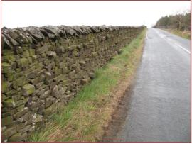
A second layer of throughs is required if the wall is around 6 feet (180 cm). The same advice given above applies to them.
