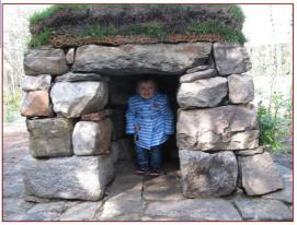
This partly underground storage area was covered over with soil and then seeded. The inside was corbelled to create a large dome.
