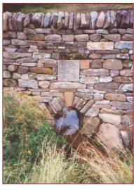
Clapper bridges are useful over water – or it is possible to use a simple arch.
